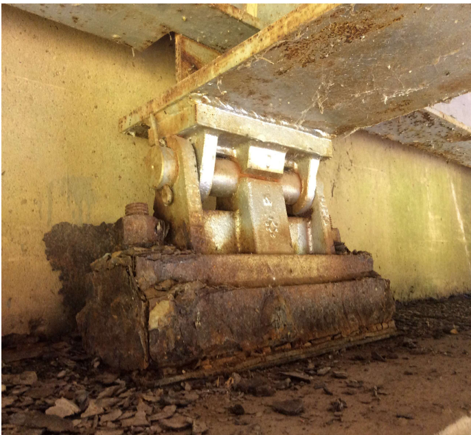
PHOTO 1 Description Rust, pack rust, and section loss to bearings.
