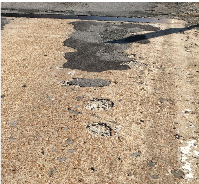
PHOTO 1 Description Several spalls and delaminated areas to deck. Unsealed cracks to deck.
