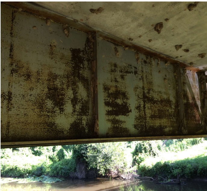
PHOTO 1 Description Paint flaking and surface rust to girders.
