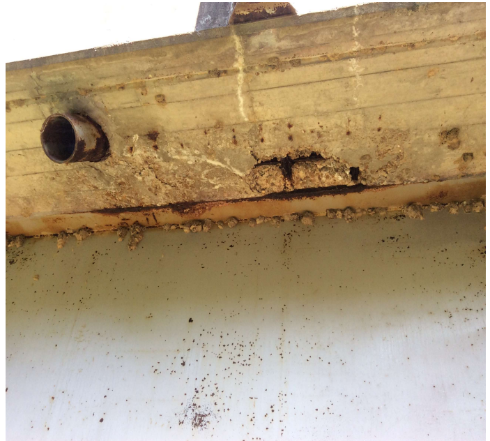
PHOTO 2 Description Spall with 2' of rebar exposed to Right overhang at end of span.
