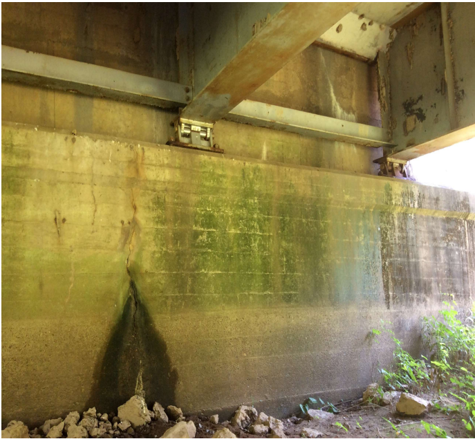
PHOTO 1 Description Full height vertical efflorescent cracks with leaching and rust stains at Abutment 2.
