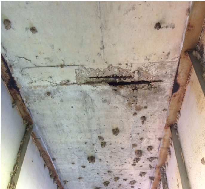
PHOTO 1 Description Spall with 3' of rebar exposed to soffit between Girders 1 and 2.
